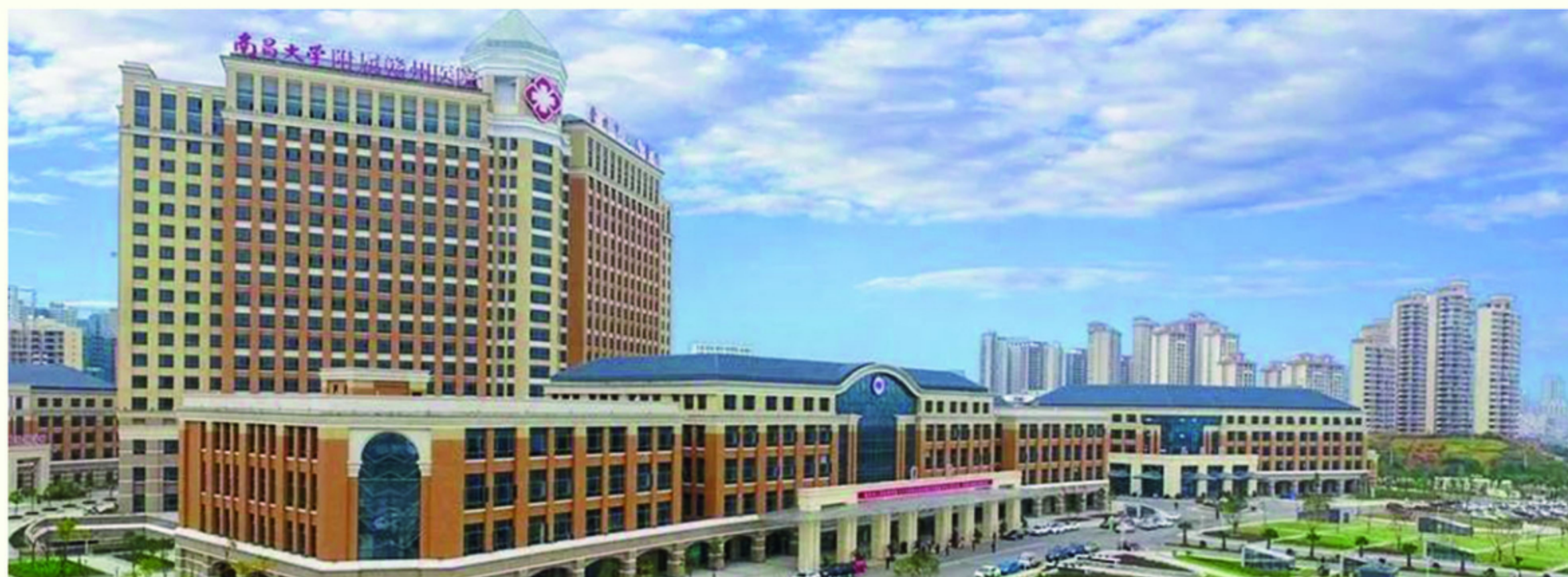
GANZHOU PEOPLE'S HOSPITAL SOUTH BRANCH
